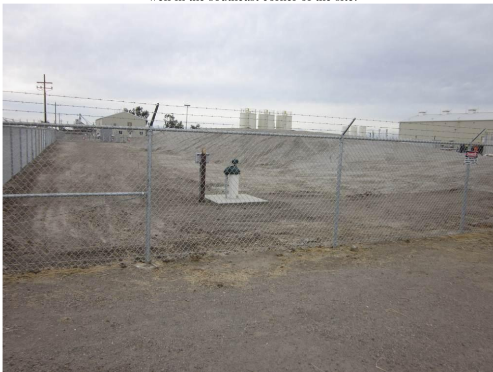
Photo 2: Two cathodic protection wells have been installed at the Compressor Station site. Pictured is the well in the northeast corner of the site.
